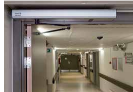
Besam swing door operators can be retrofitted to existing manual and automated doors
